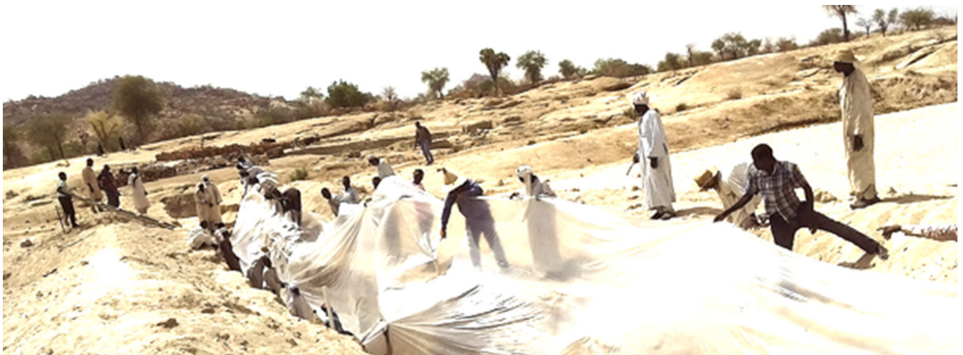
Figure 2: Placing the plastic sheet in the trench (Korlongo Bagoua-Guera-Tchad May 2019)
